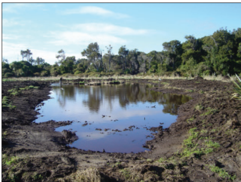
Newly excavated pond
